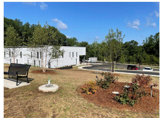
Favarr's Adaptive Wellness Center (exterior)
